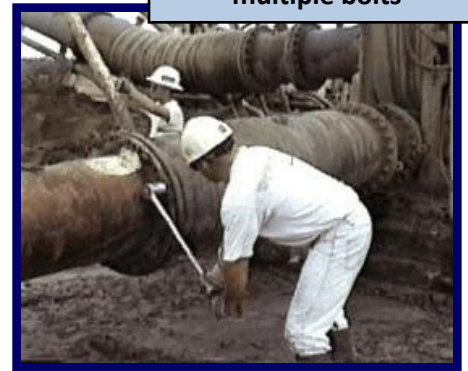
Removing /tightening multiple bolts
