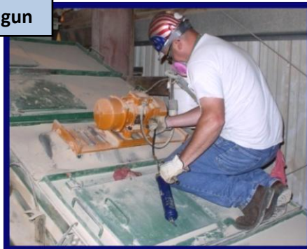
Preparing bags for sealing operation
