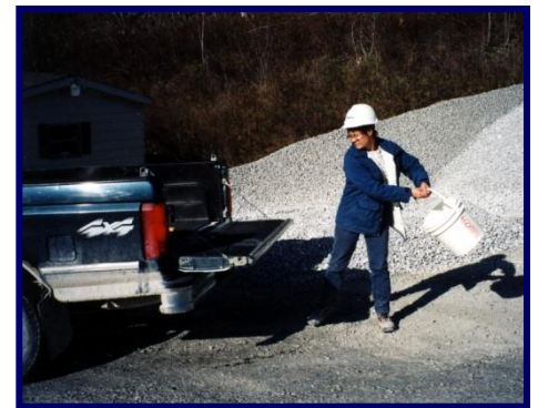
QA Tech swings sample bucket to compensate for a lack of muscle strength needed to lift the bucket into the truck.
